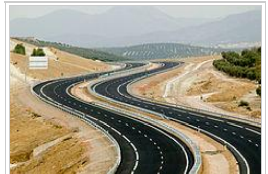
The Autovía del Olivar which unites Úbeda with Estepa in Andalucía in southern Spain. A geometric design saved on construction costs and improved visibility with the intention to reduce the likelihood of traffic incidents
